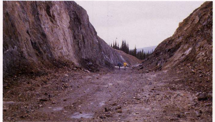
Looking east along open cut
